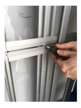
There are 6 screws for each gate and they have tamper-proof heads. An appropriate screw bit is shipped with each gate for installation of the screws. The screws are compatible with most tamper proof #10 screw drivers.
